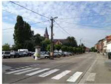
Kern Drieslinter: 'dorp plein' (parking) tegenover school
